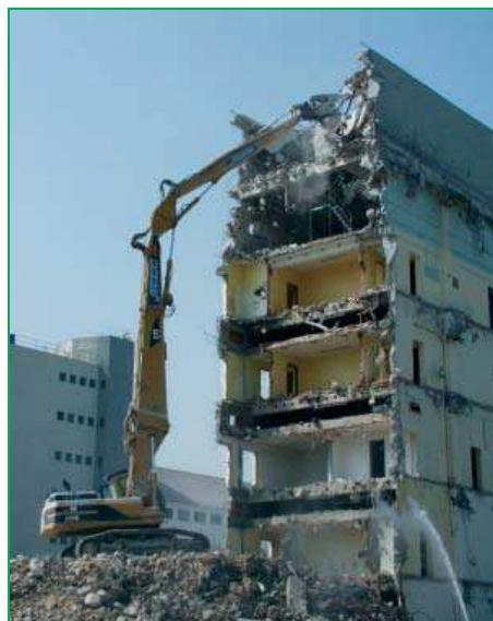
Figure 15 - Controlled deconstruction (Source: Kontrollierter Rückbau / BayLfU 2003)
